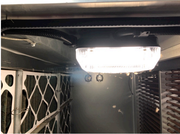
Insects within an AHU
